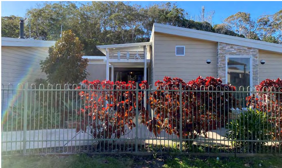
Figure 5A. Amenities building
